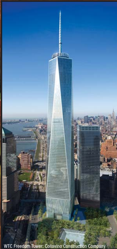
WTC Freedom Tower: Collavino Construction Company
