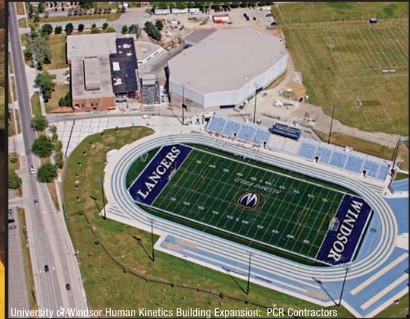
University of Windsor Human Kinetics Building Expansion: PCR Contractors
